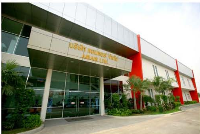
Amair Limited - Air Handling Center of Excellence
